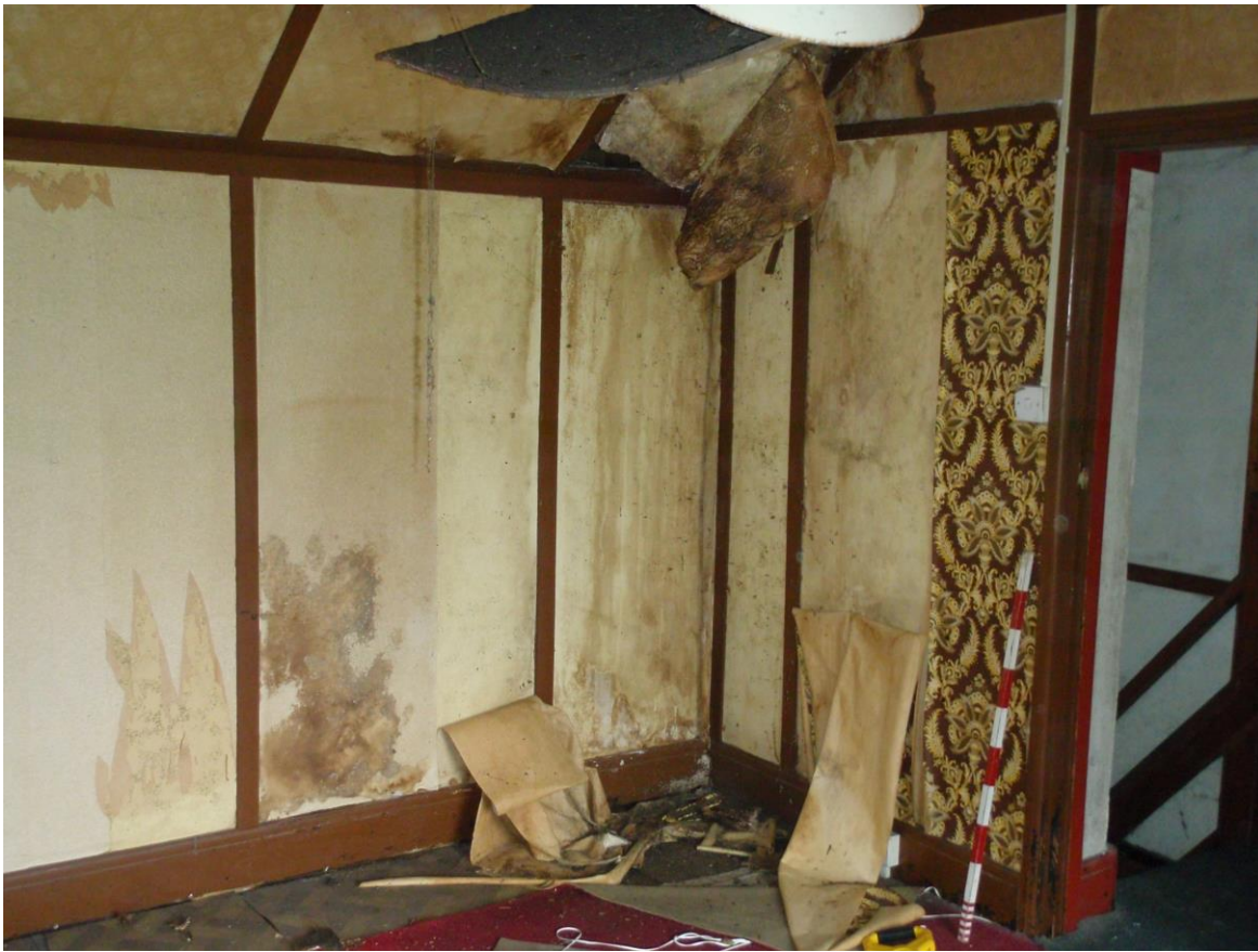
Plate 20: Upstairs Room Five looking west towards staircase and landing
