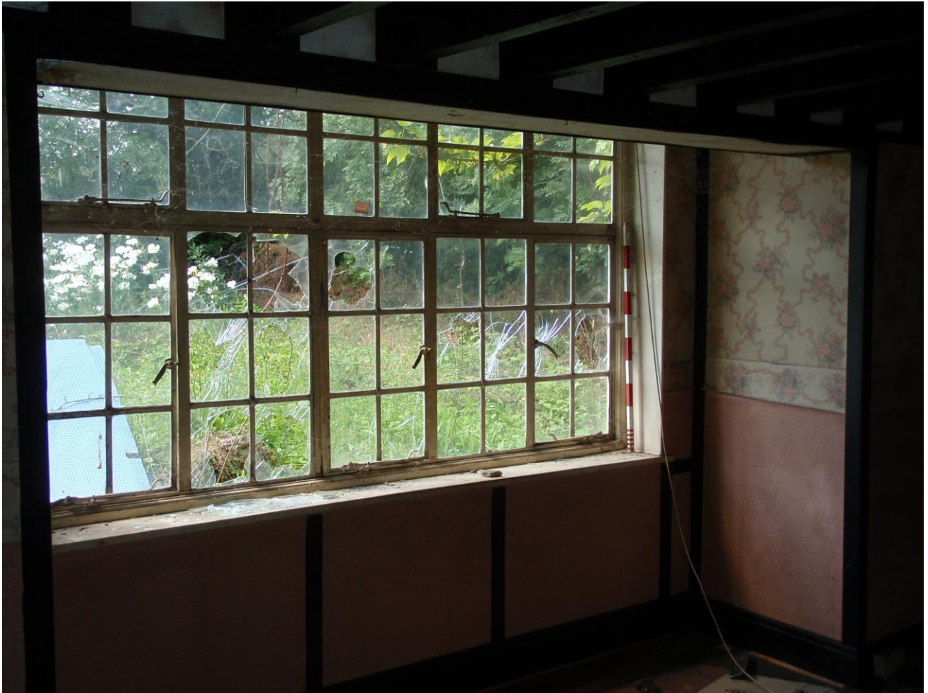
Plate 24: Window details Room Two
