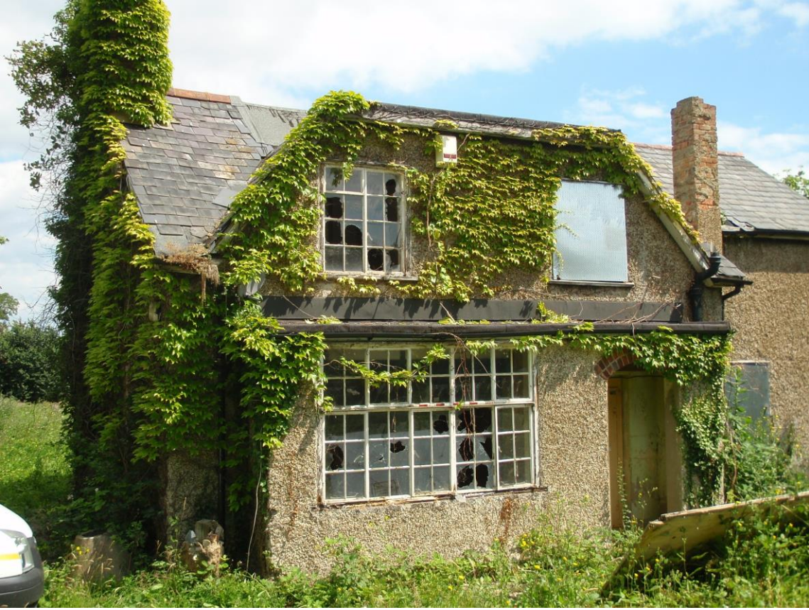
Plate 8: South elevation shutters removed
