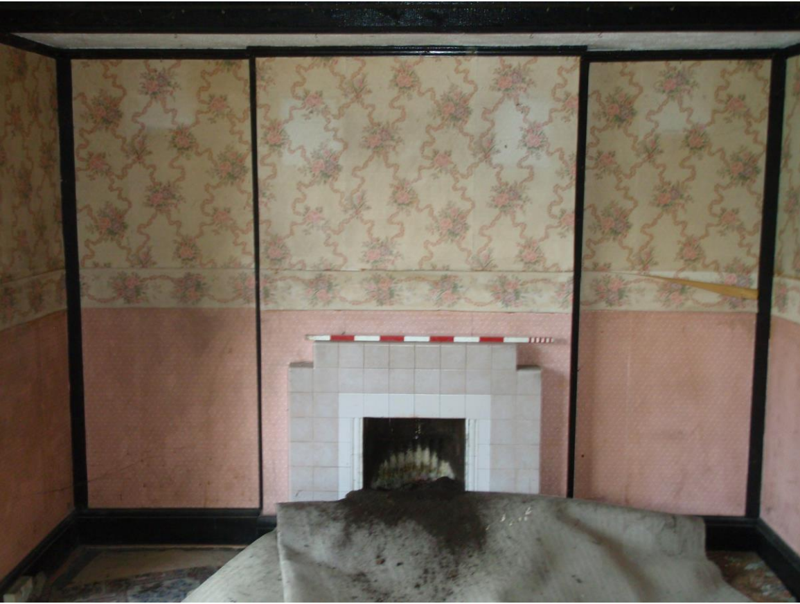
Plate 12: Room Two (looking west)
