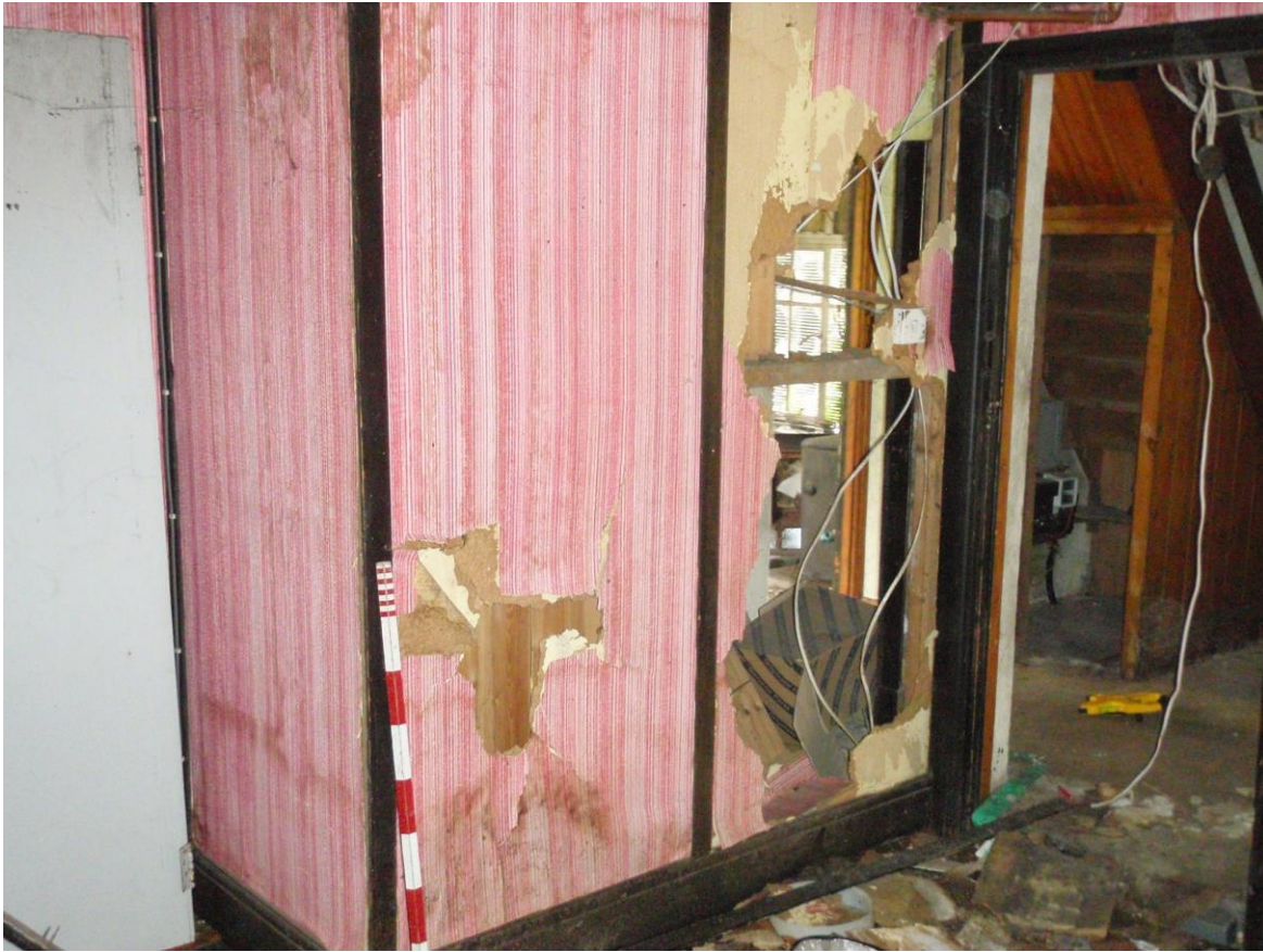
Plate 18: Room Three looking towards front door hall and staircase
