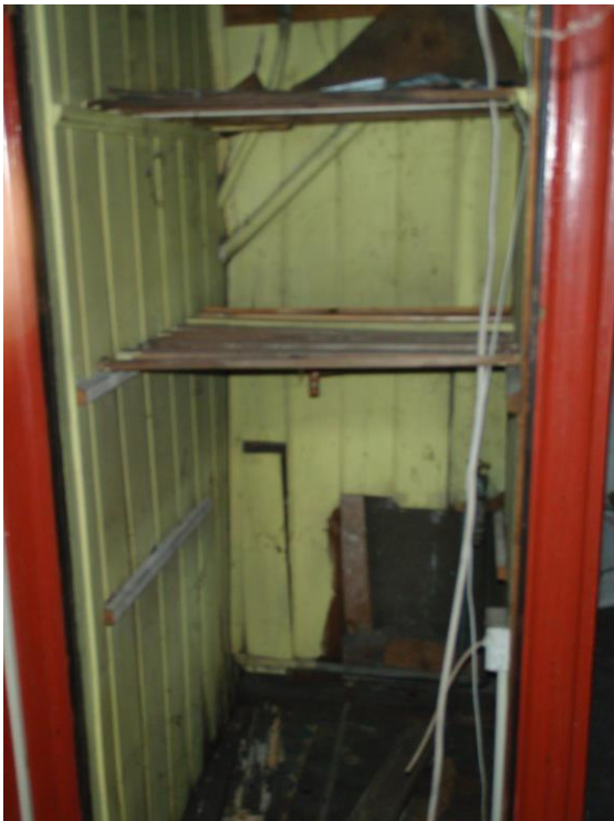
Plate 25: Airing cupboard details upstairs landing
