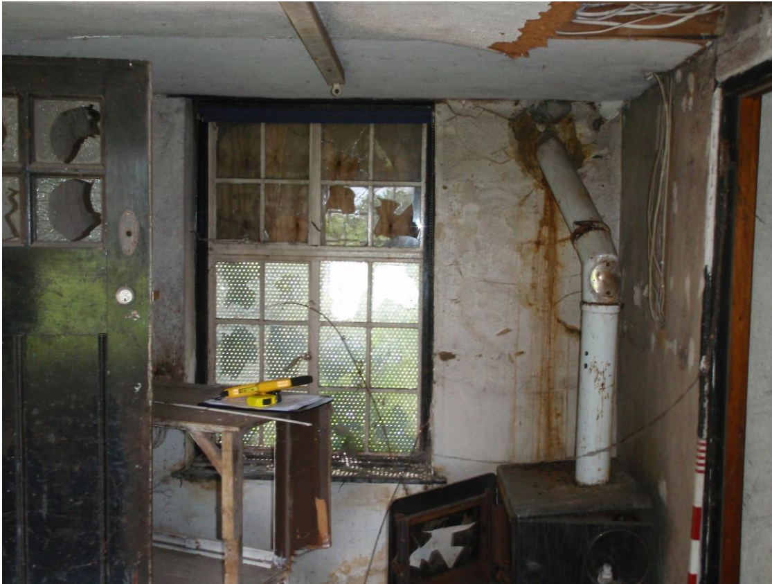
Plate 10: Room One with outside access door on left (looking SW)
