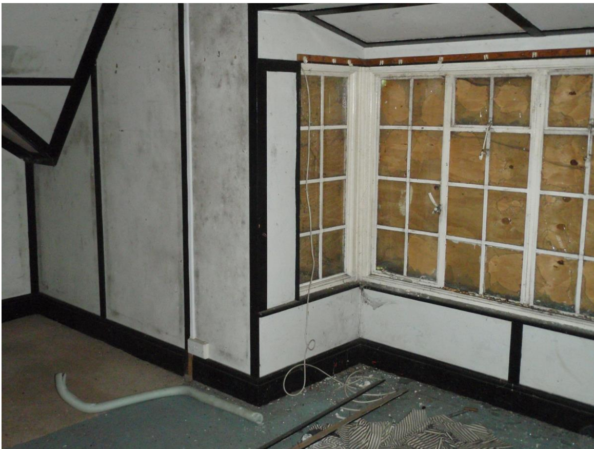
Plate 19: Room Six upstairs bedroom (looking north)
