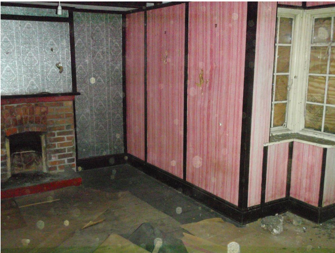
Plate 15: Room Three looking west
