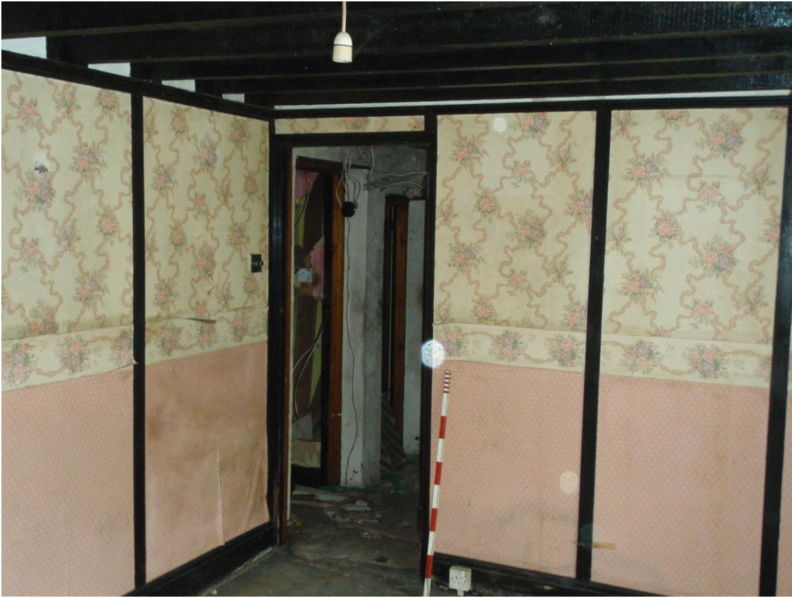
Plate 14: Room Two looking east towards front door passage and stairs. Room Three on left
