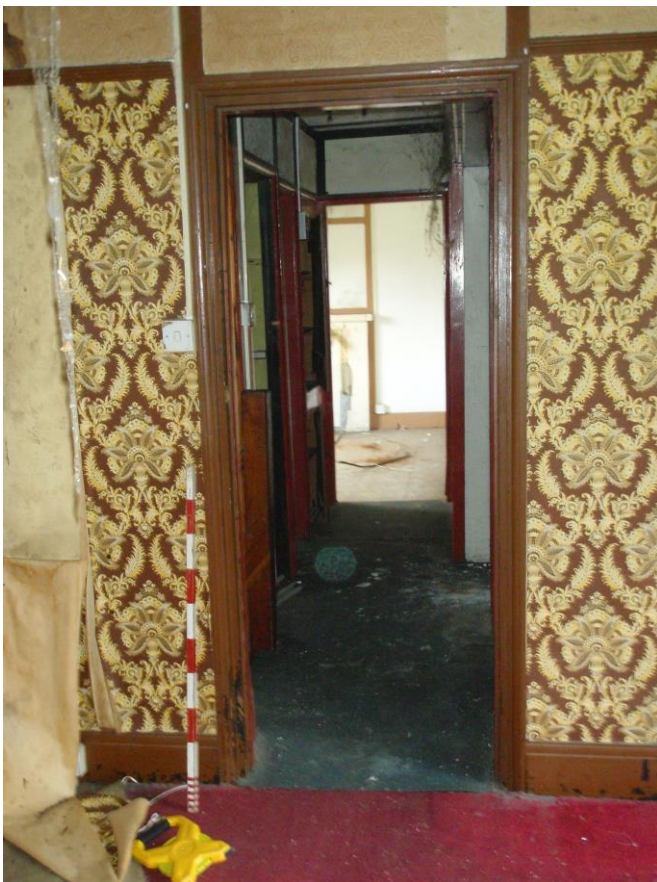
Plate 21: Room Five looking through landing to Room Four
