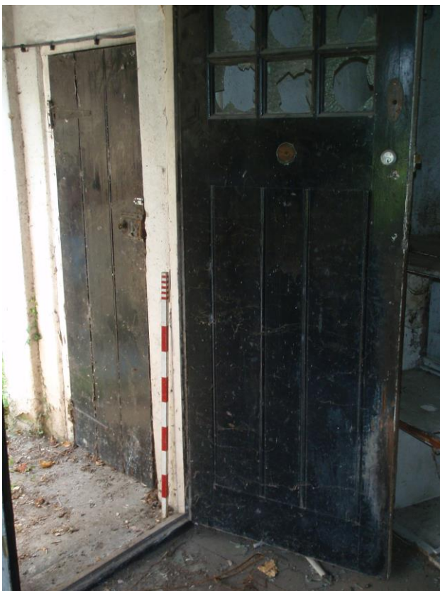
Plate 11: Side access door Room One (looking south)
