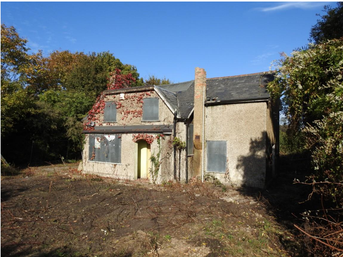
Plate 2: Southern elevation; five metre scale
