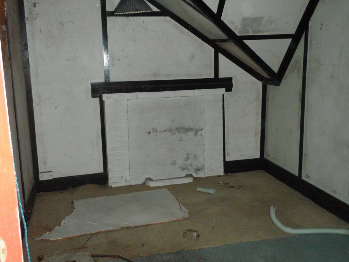
Plate 22: Room Four (looking west)
